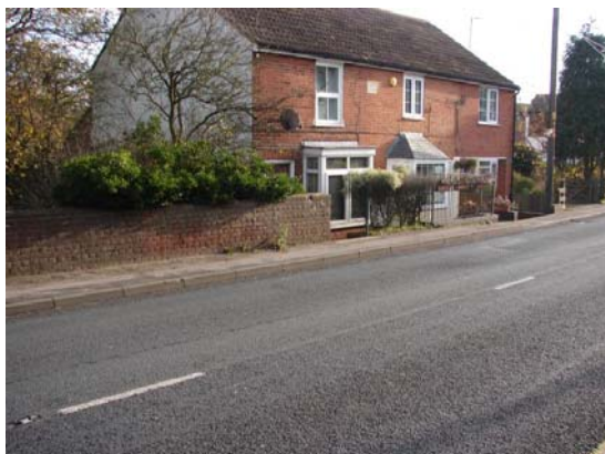
Some properties adjacent to the Blean Hill road have thresholds below road level
