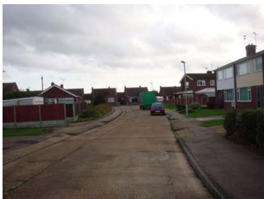
Aldridge Close in Greenhill which has an unusual raised drain and open space adjacent to the road for water storage
