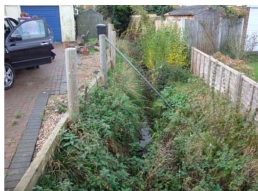
Ditch which passes under Terminus Drive in Beltinge
