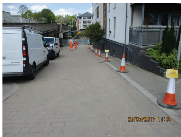
Lower site access road
