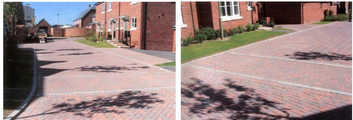
**Photos H.3 and H.4** – Permeable paving in a residential development
