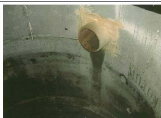
Photos A.1 and A.2 – typical examples of ring soakaways
