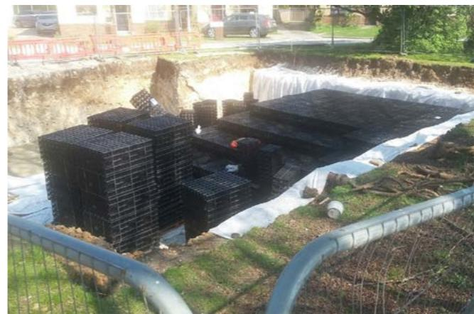
Underground attenuation and piped sections should be designed for a minimum of the 30-year rainfall event. Attenuation of events exceeding the capacity of the piped system may be achieved by temporary flooding of open spaces.
