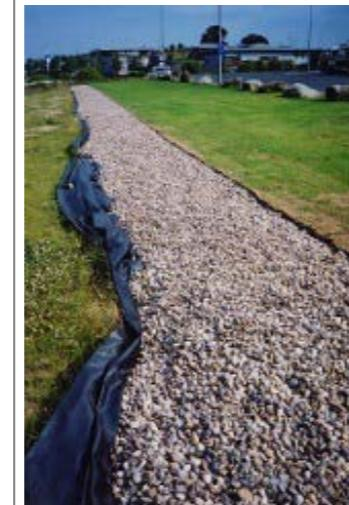
**Photos C.1 and C.2** – typical examples of filter drains, filter drain (left) Filter trench (Source: Susdrain) (right)
