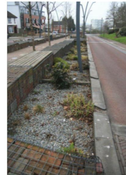
**Photo G.3** – typical example of Bioretention area (Source: Susdrain)
