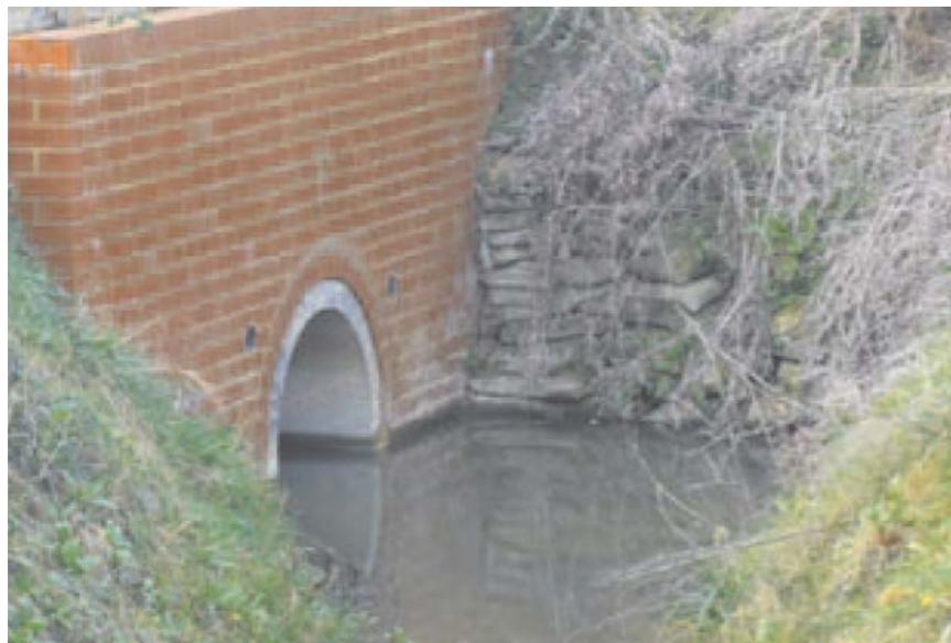
**Photo J.1** – Example of a brick headwall
