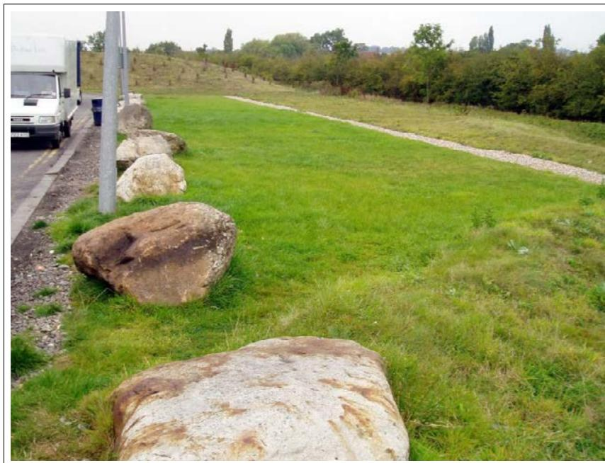
**Photos D.1** – filter strip leading to a filter drain to the right (Source: Susdrain)
