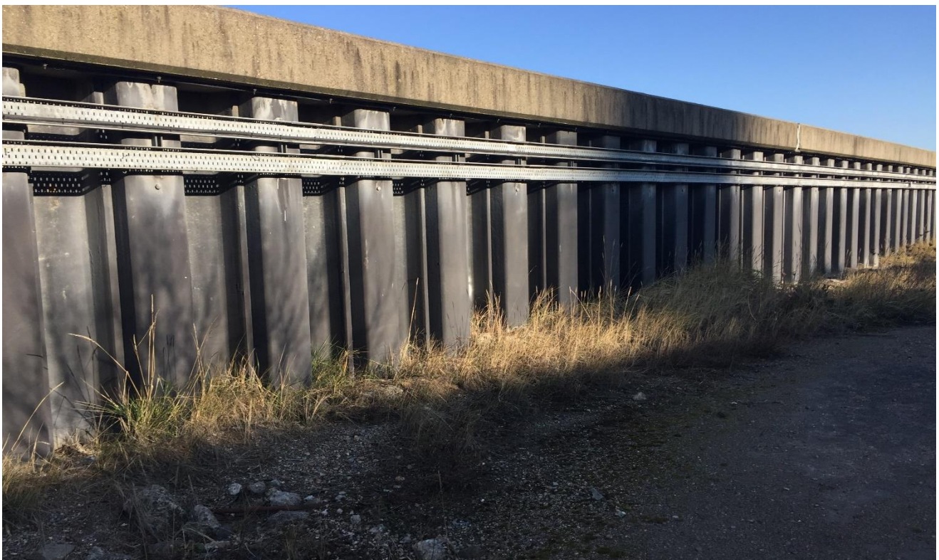
Figure 4: Tidal River Thames Defences from within Site
