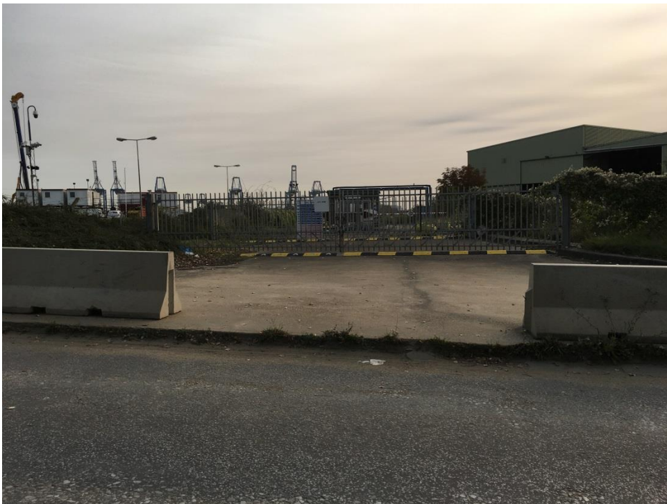
Figure 2: Unmanned Secondary Entrance
