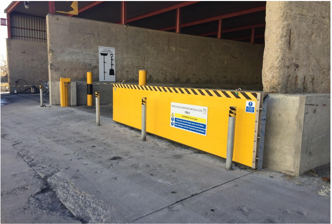
Figure 3: Example of Onsite Flood Gate
