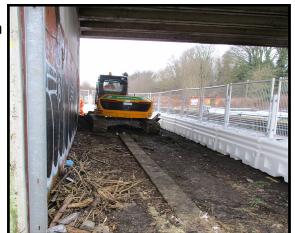
Pier 3 safely cordoned off to allow excavation
