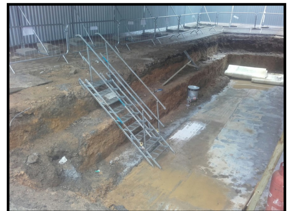
Pier 1 concrete base for temporary propping
